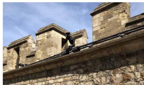
Top: GTC member Phil Nixon operating at the top of one of the historic towers Bottom: Discreetly placed tracking camera – a ROC head supplied by GTC sponsor Matt Gladstone of Cammotion
